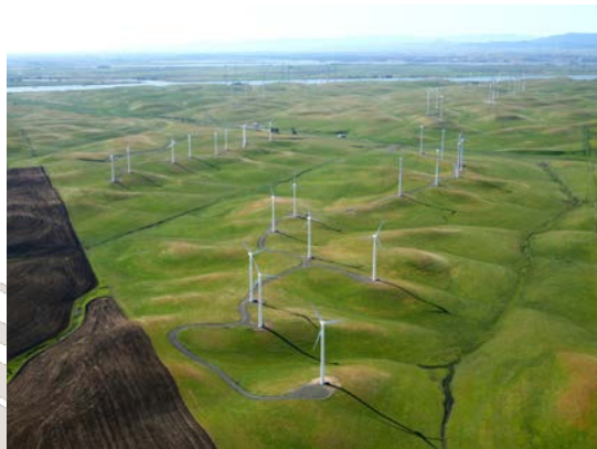
Solano Wind – 280 MW
