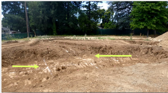
Grid soil sampling around the area where soil contaminated with lead was removed. Faint white lines show the grid pattern used for sampling.
