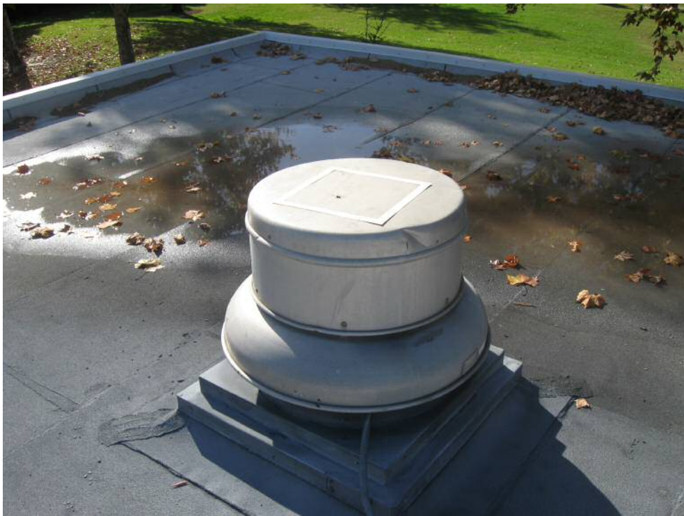
Roof above Range - sampling top surface of exhaust fan
