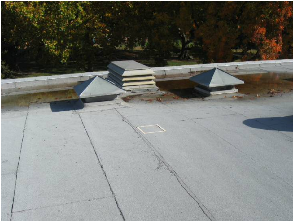
Roof - sampling surface of roof in middle of roof "field"
