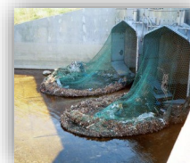
Nets/Socks Over Discharge Pipes
