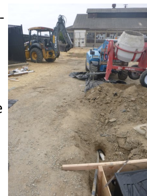
Soil Vapor Extraction pipe approach begins far from the affected building to achieve the necessary gradual descent angle.
